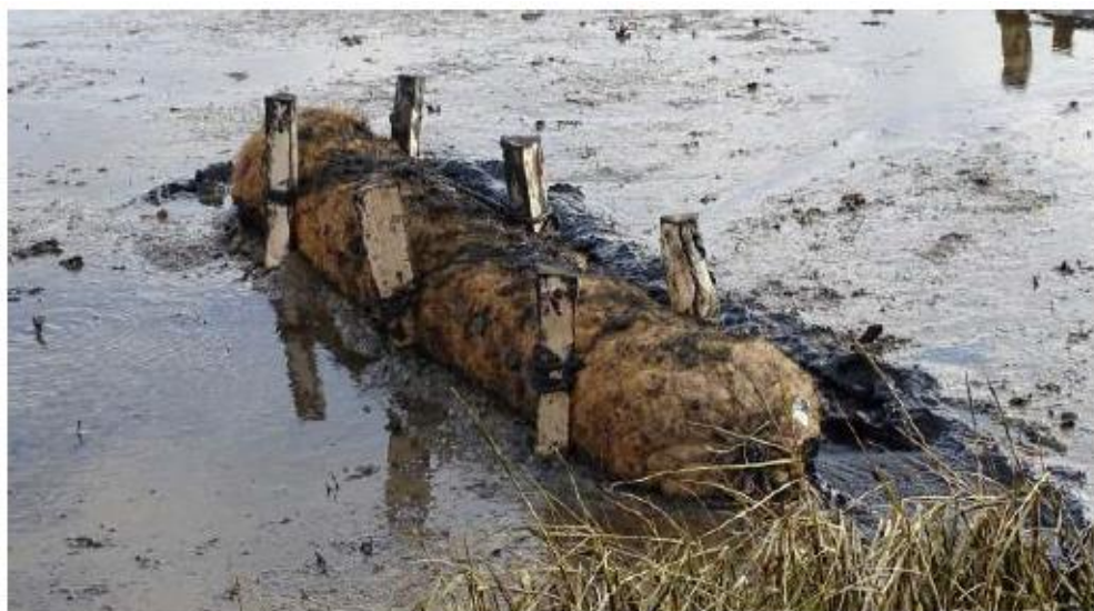
Figure 7-1 Typical Coir Roll installation
