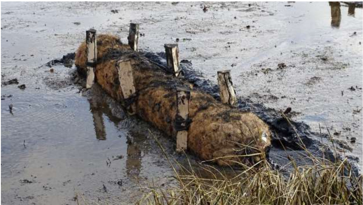
Figure 2. Newly installed coir role to encourage sedimentation and saltmarsh colonisation
